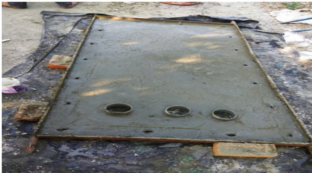
Panels with Bamboo Reinforcement.
